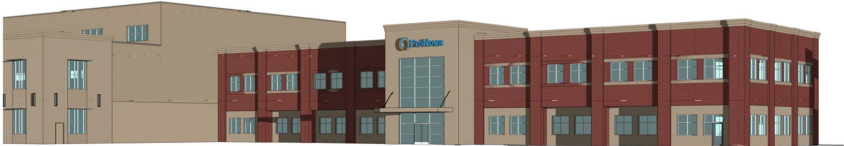
OFFICE BLDG (VIEW FROM NW)
