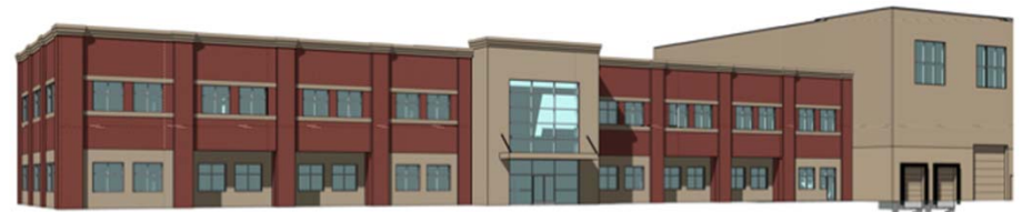
OFFICE BLDG (VIEW FROM SW)
